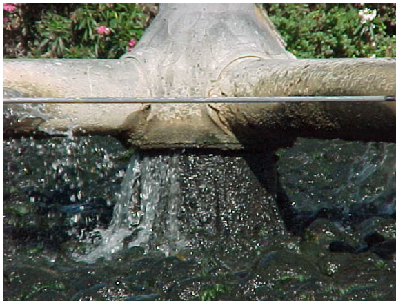
Water pouring out of bottom of main drive. No replacement parts available due to age of equipment.
