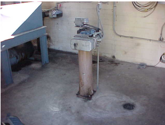
Recirculation valves are obsolete for parts. These were the valves installed in 1989 and need to be updated.
